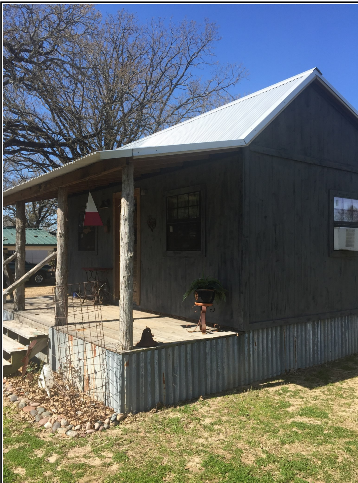
Jody and Bob's historical home restoration.
