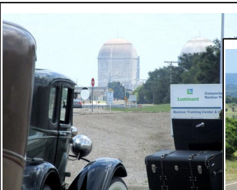
Comanche Peak Nuclear Power Plant
